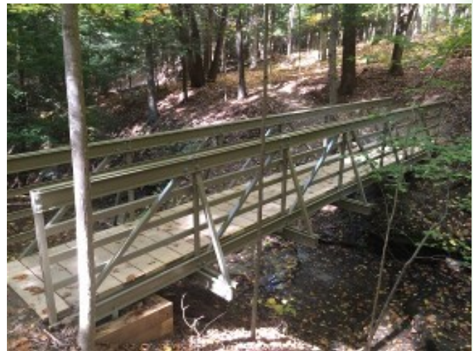
Fiberglass bridge on Rob's Trail.
